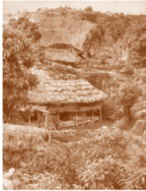
Houses typical of the hills.
