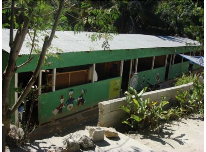
Example of a TLS in Haiti made out wood by an International Humanitarian Organization
