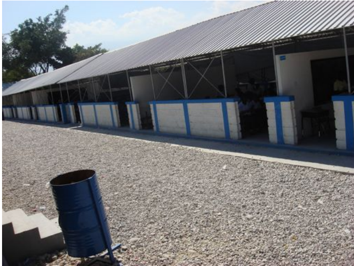
Example of a TLS in Haiti made out of concrete blocks and metal sheets
